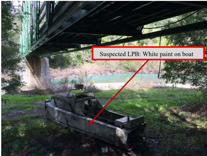
Figure 14. Lead-Based Paint Sampling Locations
