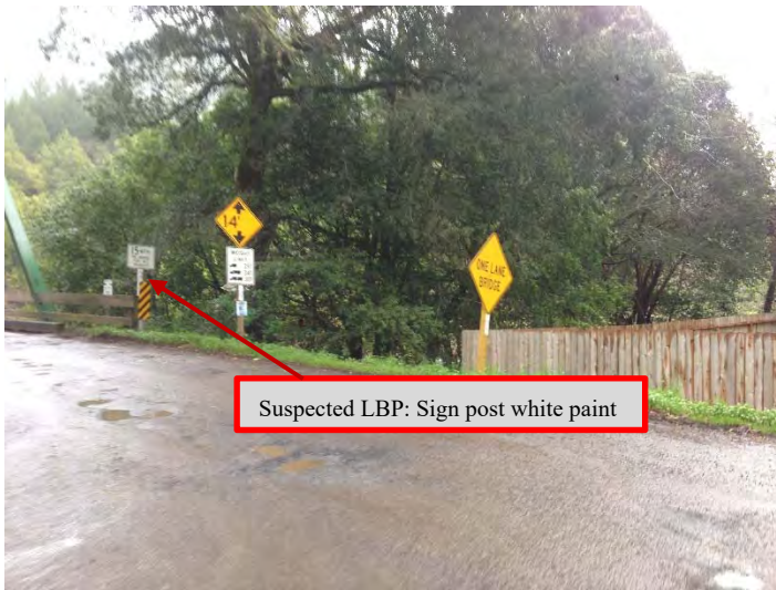
Figure 13. Lead-Based Paint Sampling Locations
