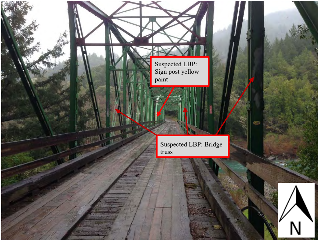
Figure 12. Lead-Based Paint Sampling Locations
