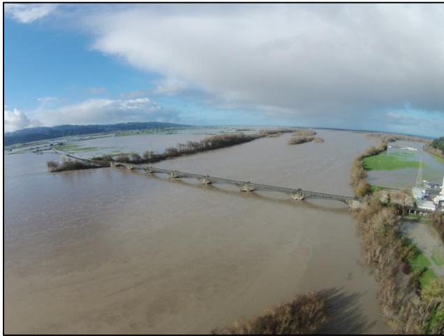
Photo 1. Eel River Flood January 11, 2017, looking to the southwest. Fernbridge in foreground.
