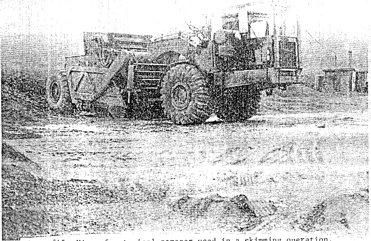
Photo #15 - View of a typical scraper used in a skimming operation.
