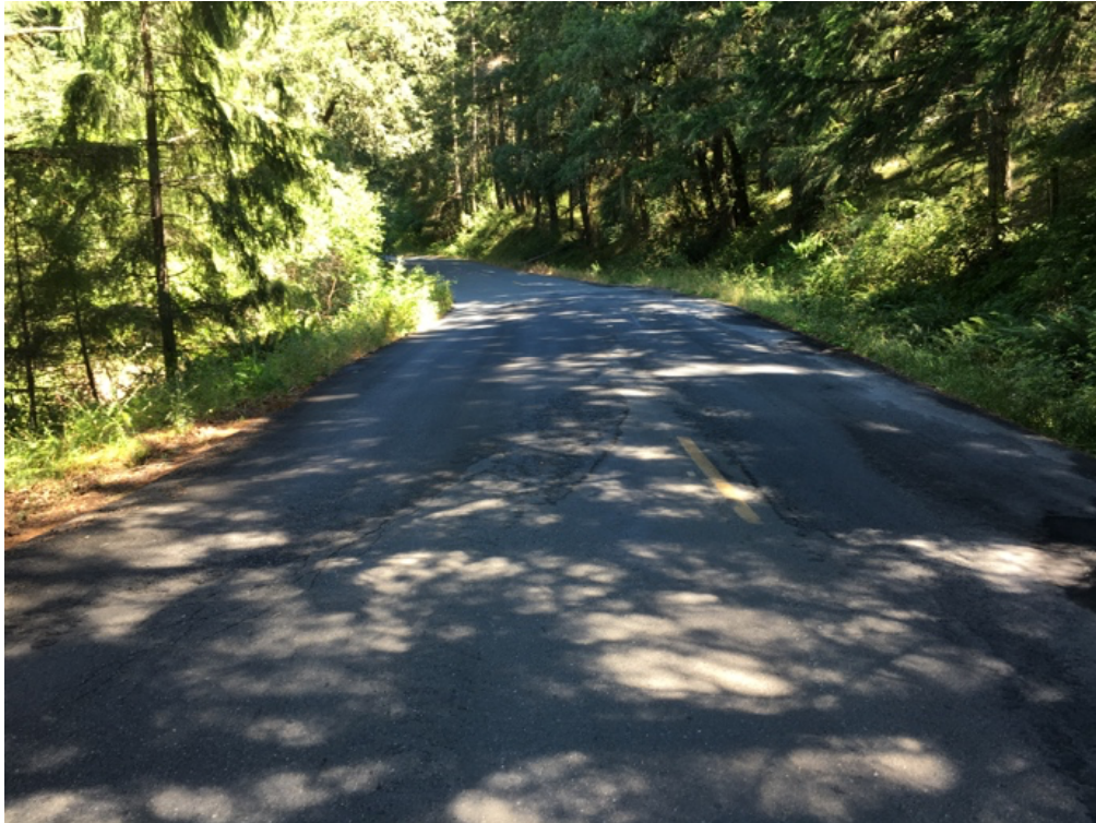
Photo 5 – Looking Northeast at PM 42.25 (July 2019)
