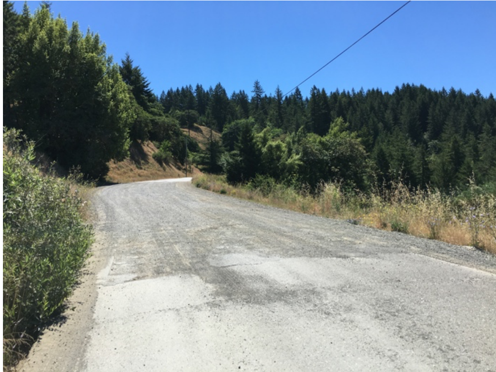
Photo 4 – Looking Southeast at PM 42.10 (July 2019)
