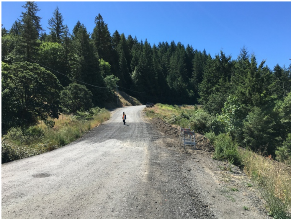
Photo 2 – Looking Southeast at PM 42.00 (July 2019)
