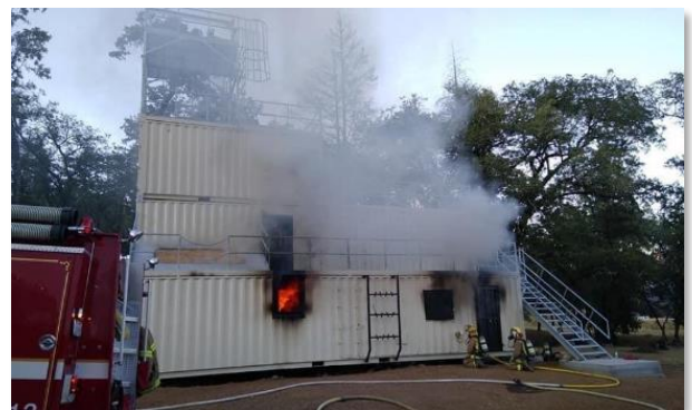
New fire training tower in Redway provided by Measure Z.
