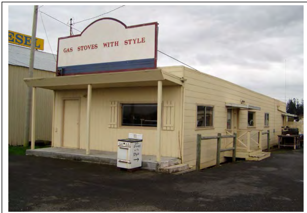
Photograph 3. 3360 Jacobs Avenue, camera facing northeast, February 18, 2002.
