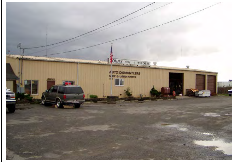
Photograph 2. Corrugated metal shed addition, camera facing southeast, February 18, 2003.
