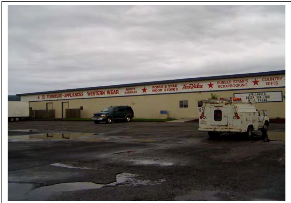
Photograph 2. View of front façade, camera facing southeast, February 18, 2003.
