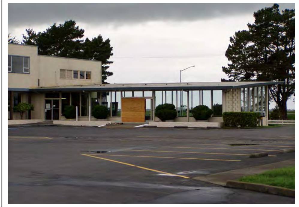
Photograph 2. Small wing on the northwest side, camera facing southwest, February 18, 2003.
