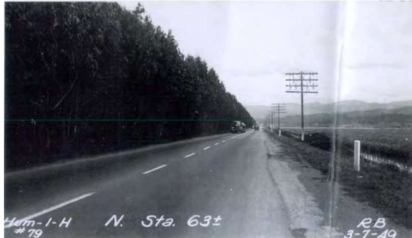
Figure 5. Highway 101 circa 1947, looking north from the current airport. Courtesy of Caltrans District 1 Photo Archive.
