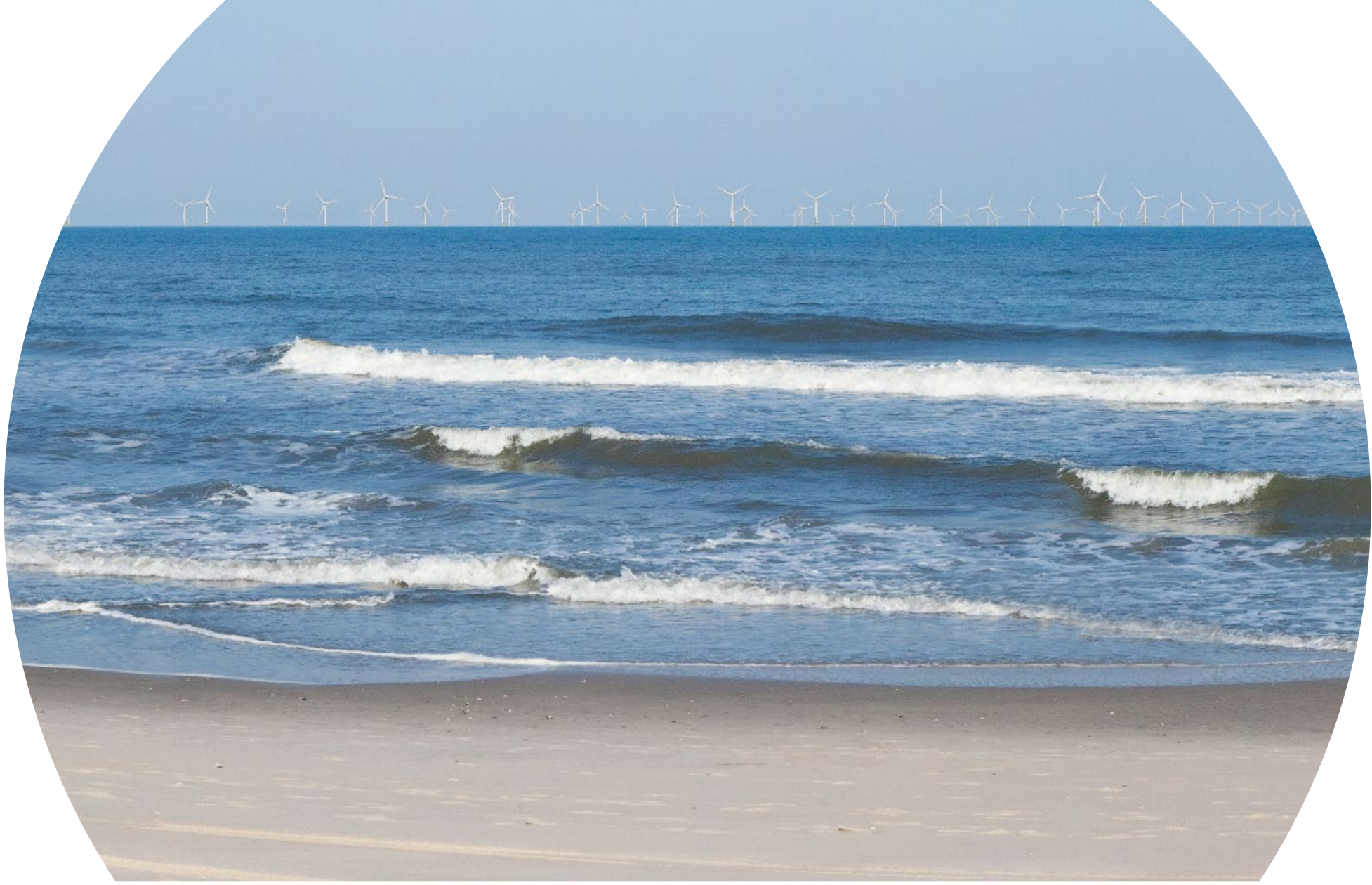
121 Turbines at 8 Miles Offshore
